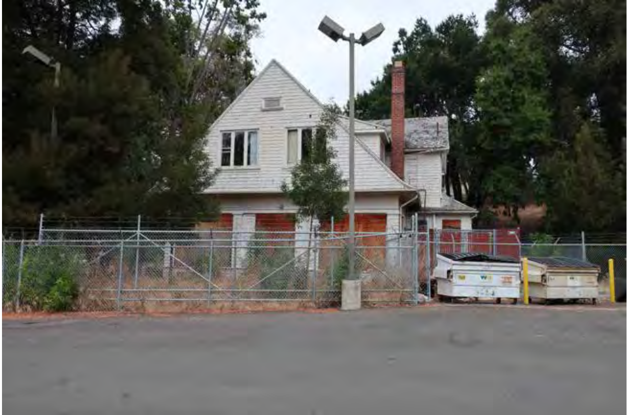
Fig.1 – Superintendent's Residence/Whitecotton Cottage, Front (south), 2018
