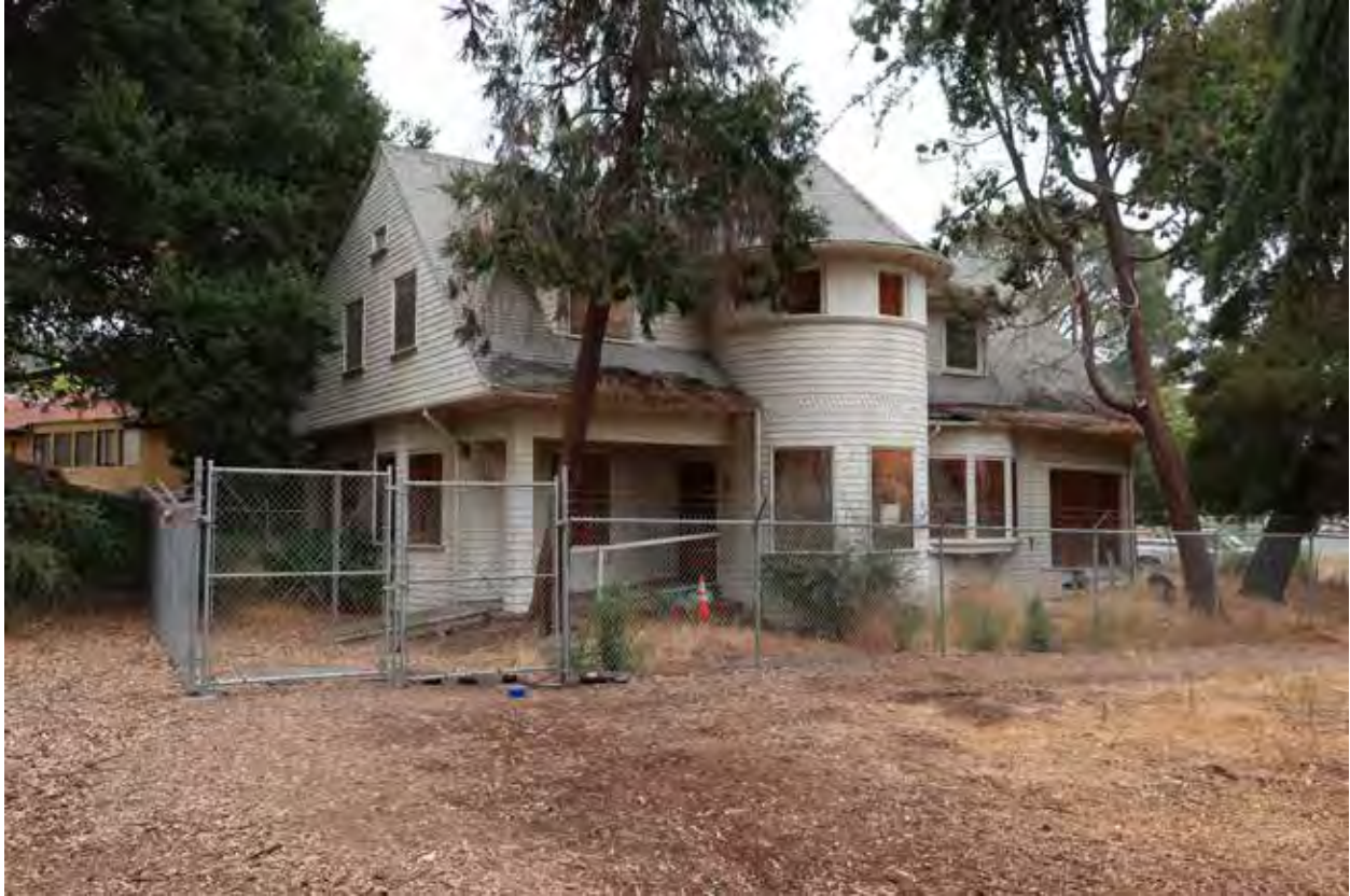
Fig.3 – Superintendent's Residence/Whitecotton Cottage, West side, 2018
