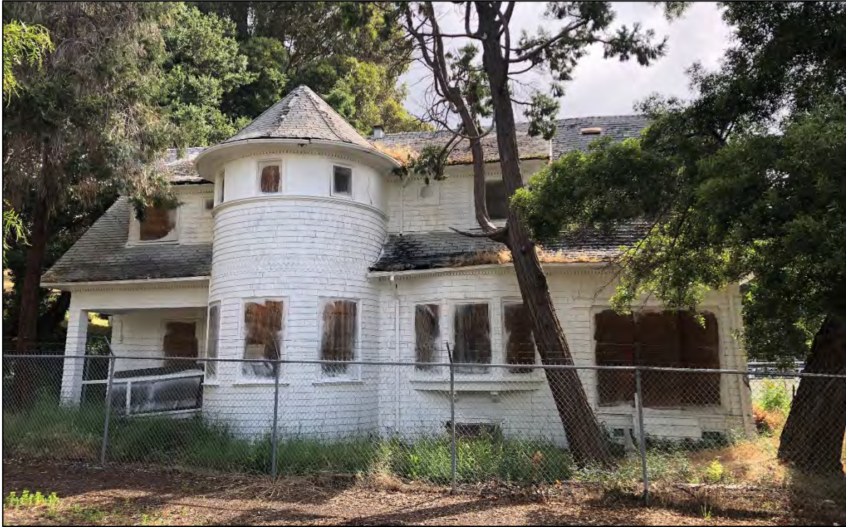
Photograph 3. West façade of Whitecotton Cottage , looking east
