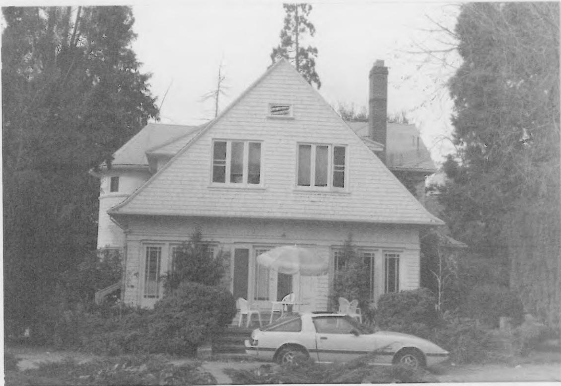
Figure 3. South Elevation, Superintendent's Residence, Fairmont Hospital.
