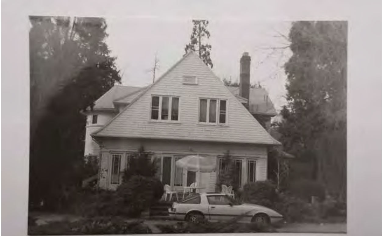
Figure 3. South Elevation, Superintendent's Residence, Fairmont Hospital.
